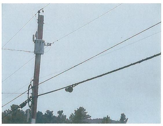
ORFORD NH POLE FP 98 PSNH 41/90 State Route 10 Photo 4 of 4 10/12/2012 T Parssinen Span to next pole shows NHOS strand crossing segTEL cable with no cable guard or other protection to avoid damage.
