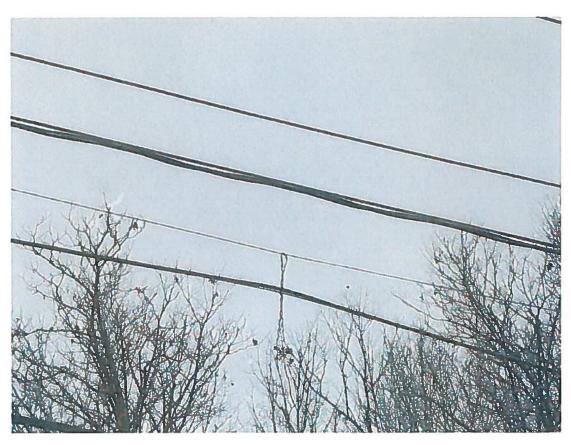
SUNAPEE NH POLE FP 17 ELCO 21 (vicinity) Springfield Rd Photo 2 of 5 11/26/2012 T Parssinen Shows device attached to segTEL fiber, pulling and bending the fiber optic cable. The top of the device is hanging from NHOS messenger strand.
